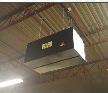
The SO 2000-I is ideally mounted underneath a ceiling but can also be placed on top of flat surfaces such as tables and desks.
