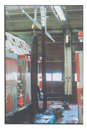
Sourcetec non-exhaust rail system series "EMNE" is specifically designed with a special pneumatic bladder for a quick unhindered release for moving and emergency vehicles. The pneumatic bladder slides onto the exhaust pipe of the vehicle, where a manual fill valve inflates the bladder for a 100% sealed fit.
