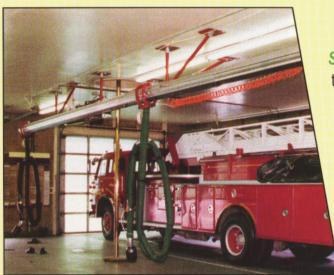
**Sourcetec** offers three types of rail systems that allow vehicles to be driven in and out of the base station while remaining attached to the exhaust removal system.
