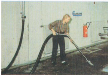
6 Vacuum cleaning equipment, complete with independent separator/dust container, can be plugged into any outlet. A complete choice of cleaning nozzles are available.
